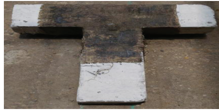
Fig. 5. Basalt fabric wrapped beam column joint
